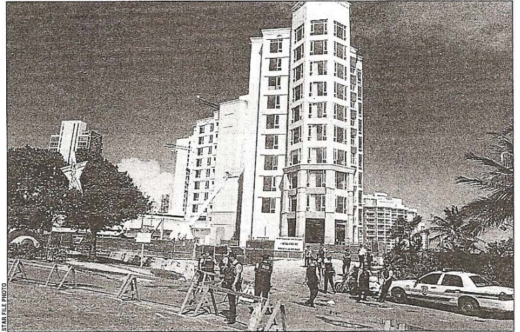
The Paseo Caribe development site in Puerta de Tierra
